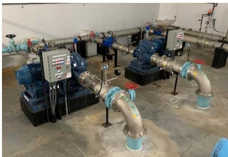
The two high lift pumps provide redundant pumping capacity into the AASWSS. The Aylmer pumps are equipped with variable frequency drives (VFD) with each pump having a rated capacity of 130L/sec. With the current VFDs being utilized as soft and stop variable frequency drives.
