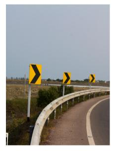
The Township of Malahide requested the installation of guard rails on Imperial Road in the Village of Port Bruce. In response, Council instructed staff to install Chevron alignment signs on the road instead, based on the Ontario Traffic Manual, along the horizontal roadway curve immediately north of Rush Creek Line.
