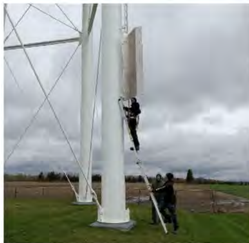
Picture - 1: Ladder Access To Tank
